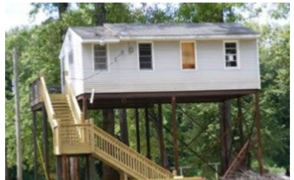
An elevated cabin in Jersey County
