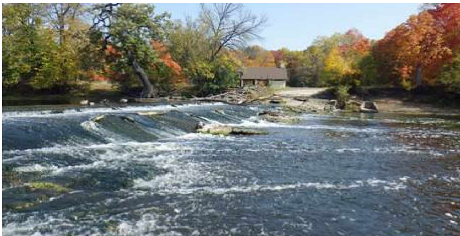
Dam 1 on the Des Plaines River
