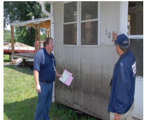
Observing a high water mark on a home.
