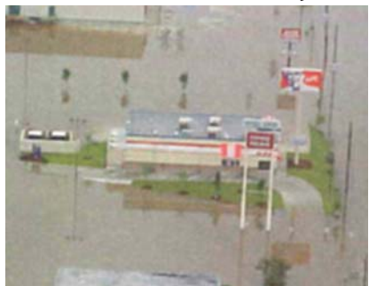
Commercial building elevated on fill be either elevated or flood proofed.
