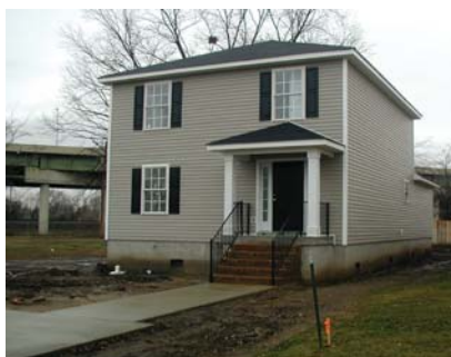
Residence elevated on crawlspace. [Note openings close to the ground to allow floodwaters to flow through and not place pressure on the walls.]
