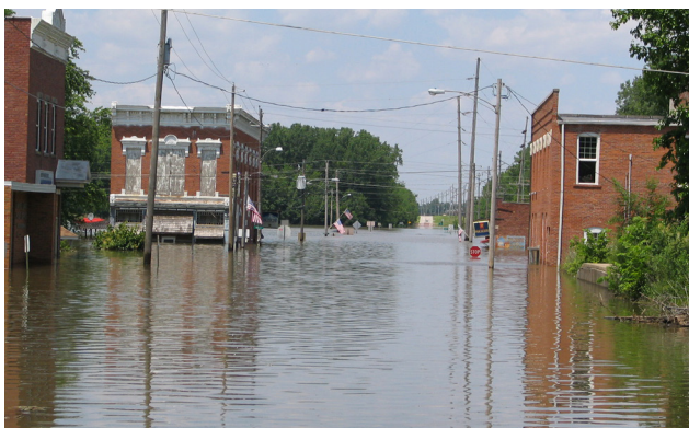
Flooding in downtown Keithsburg, prior to mitigation efforts
