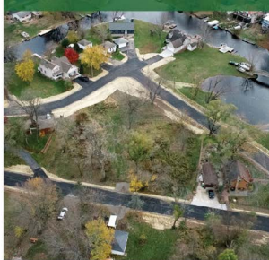
Knollwood Subdivision Flood Control Village of Fox Lake
