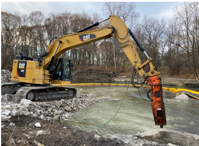
Touhy Ave Dam Removal – photo courtesy IDNR
