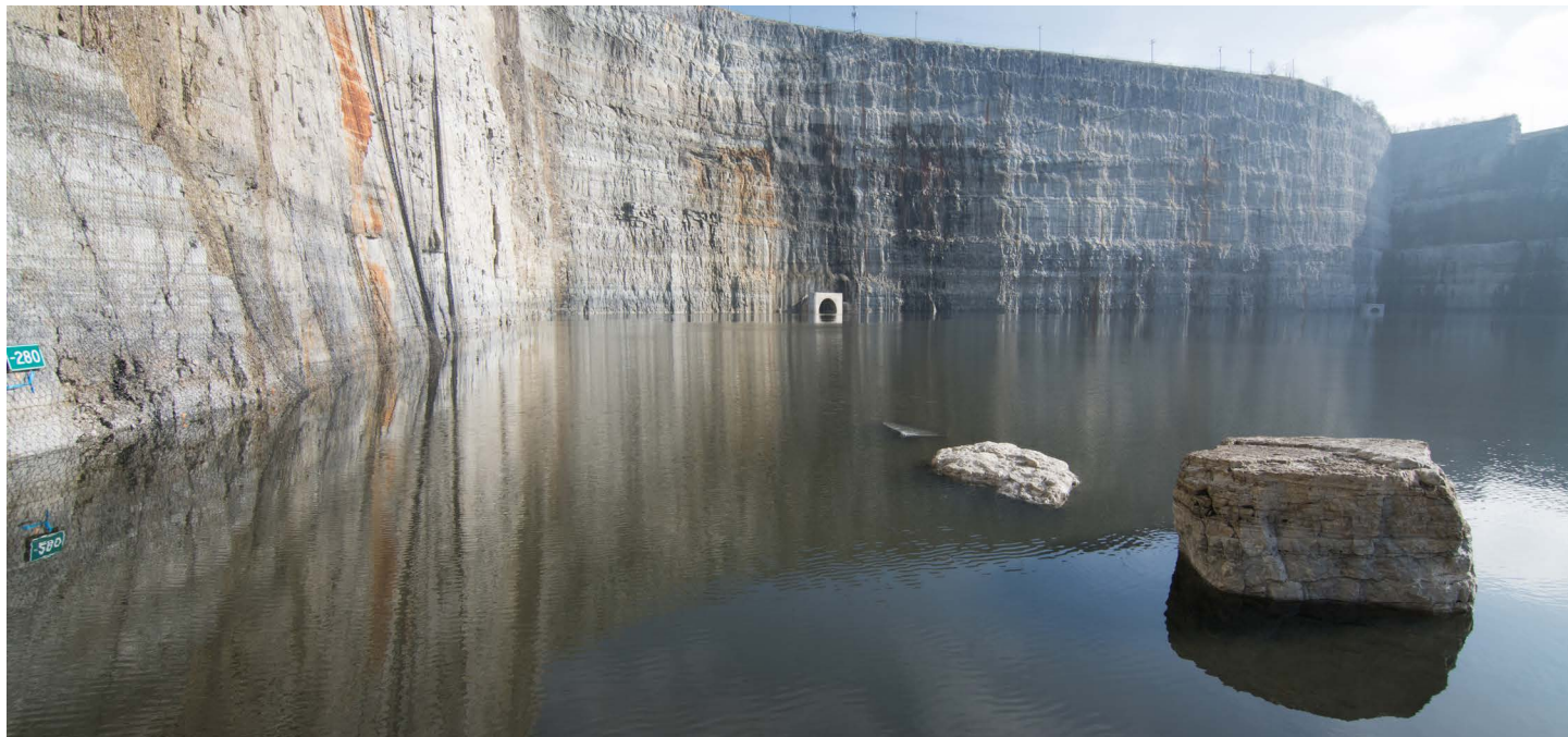
Water rises along the limestone walls of the Thornton Composite Reservoir in South Holland, a former quarry transformed into a critical component of MWRD's Tunnel and Reservoir Plan.
