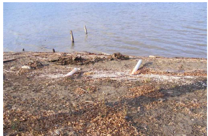
Septic field in floodplain with pipe outlet at river.
