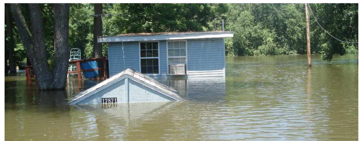
Before and After photos showing flooding at one of the repetitive loss federal lease cabins in southern Illinois.
