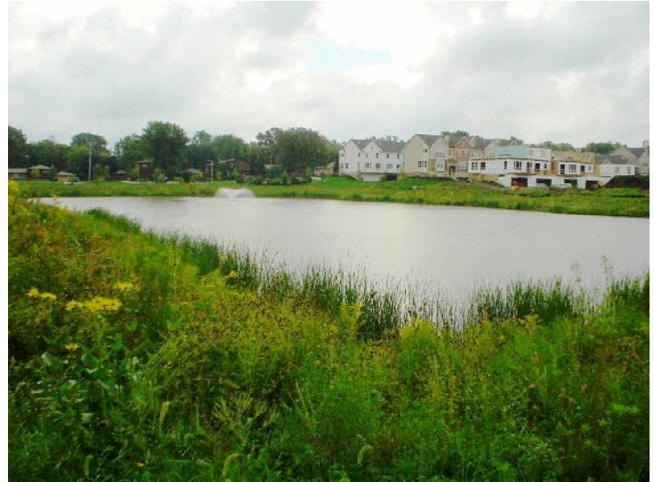
A stormwater management facility in a development built to comply with stormwater and floodplain regulations
