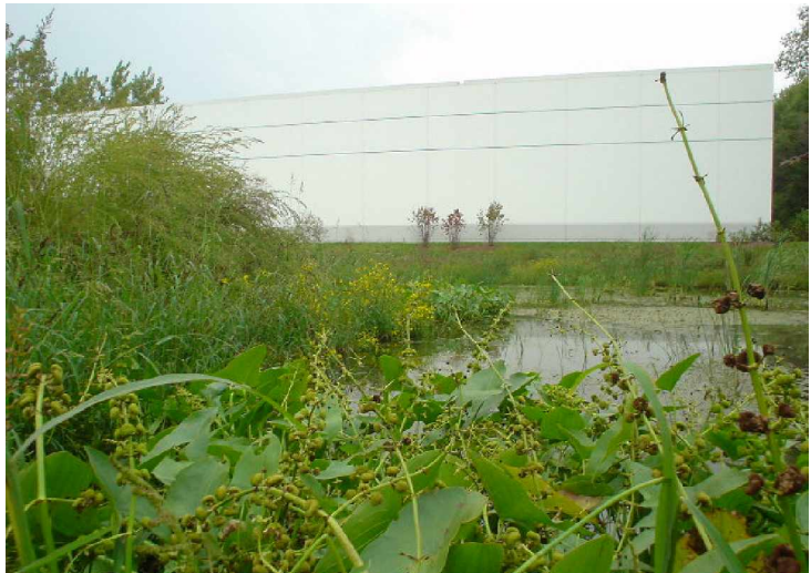
The cost to comply with regulations and build stormwater facilities is far less than damage or mitigation costs.
