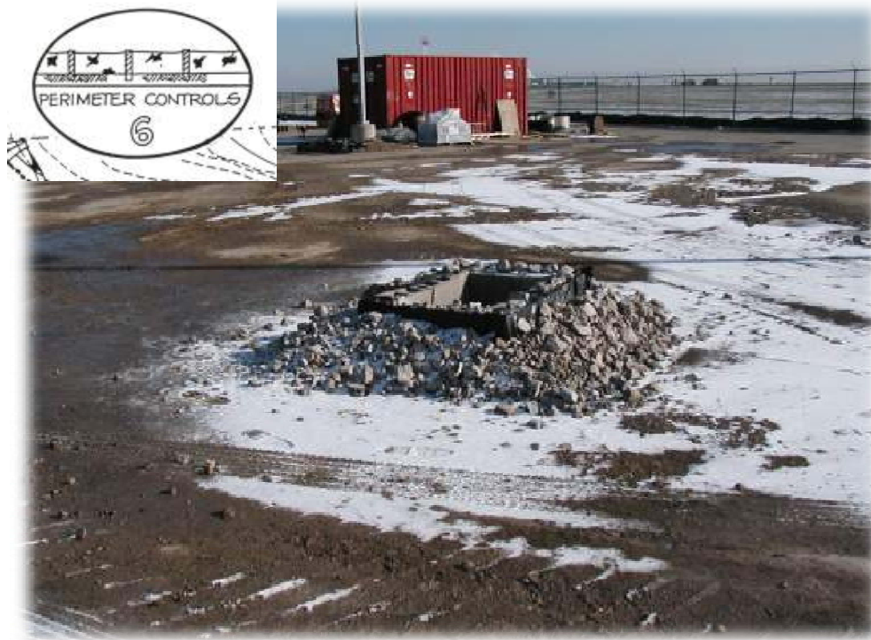
Block & Gravel Inlet Protection
