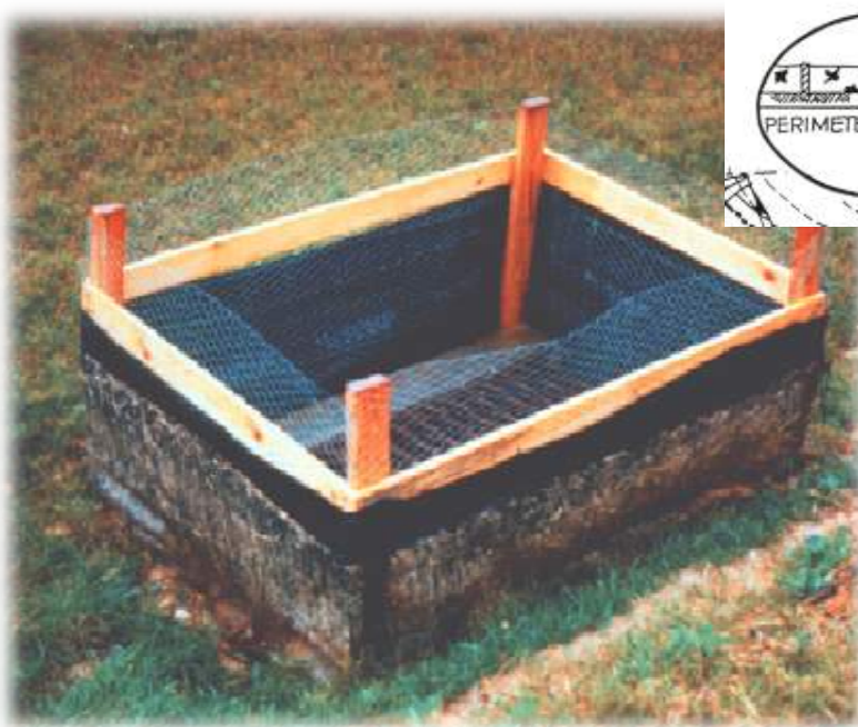
Field/Yard Inlet Protection
