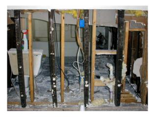
Figure 16-11: Even standing floodwater can cause substantial damage.
