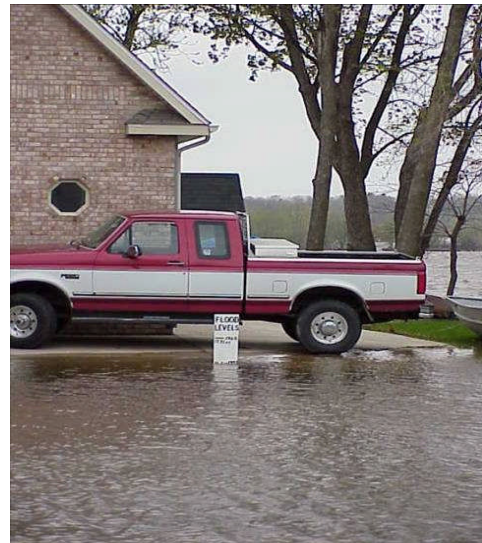
Figure 12-2: This building was elevated on fill and was not damaged by this flood.
