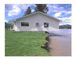
Figure 1-5: Riverine erosion can undercut structures
