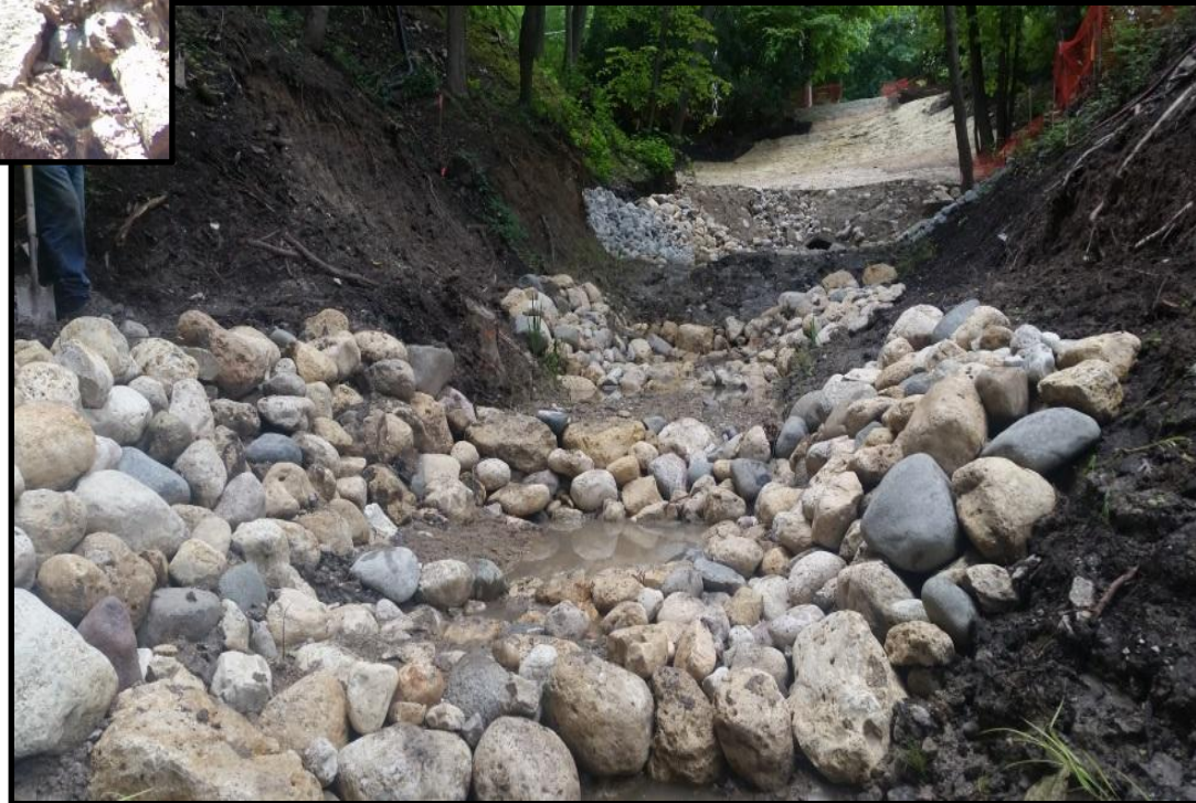
Restored Plunge Pool Outfall (After)
