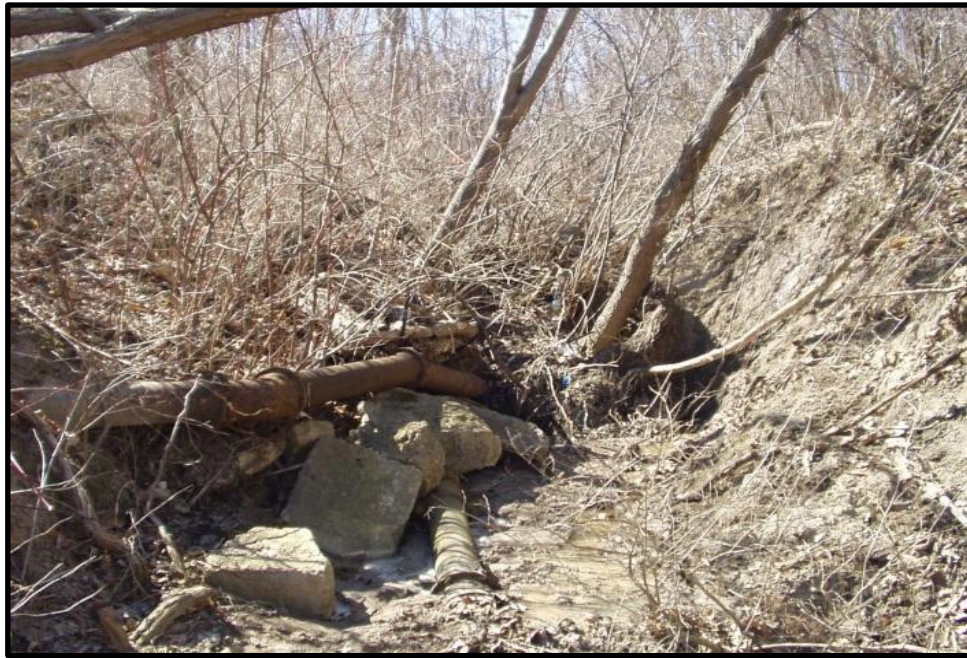
Collapsed Ravine Toe/ Distressed Utility Lines (Before)
