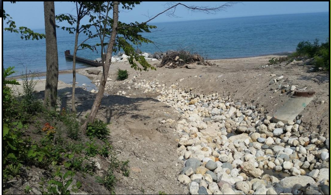
Armored Step-Up Pool/ Ravine Toe (After)
