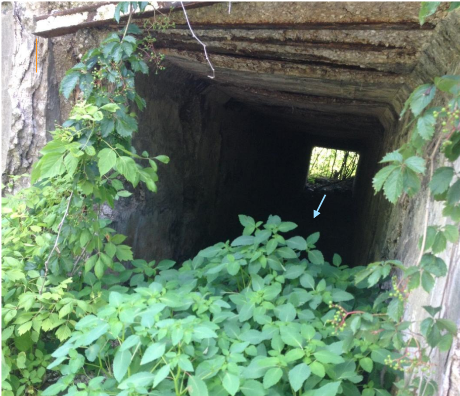
3 Lateral Box Culvert (6'X7') (Rating Curves were Developed to analyze flow through this culvert)
