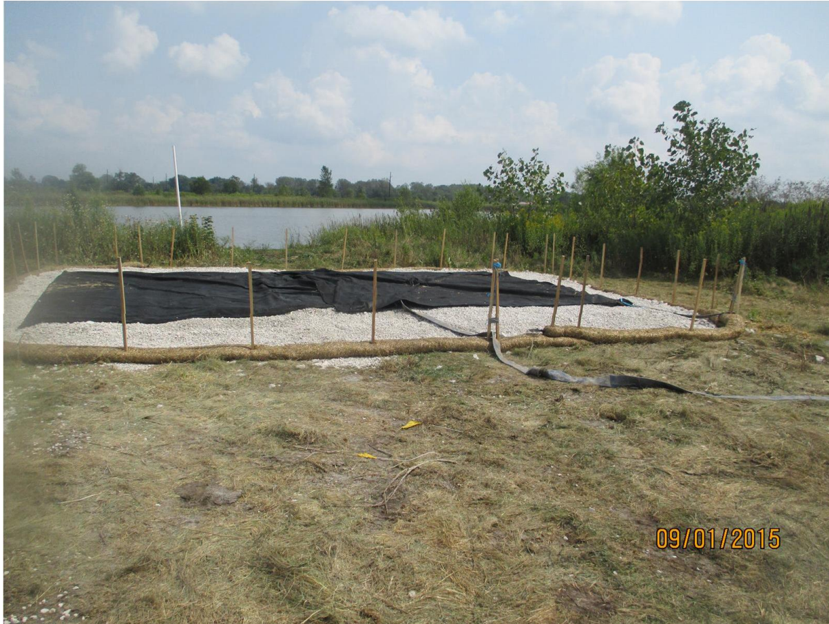
Pond dewatering – discharging into east basin
