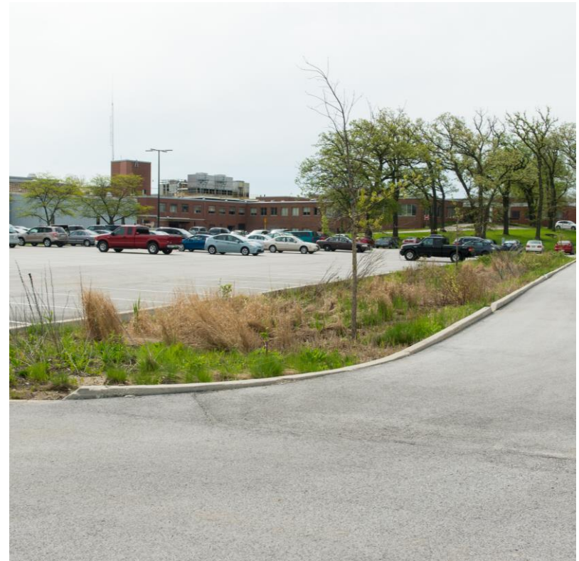
Bioswale in Large Parking Lot Manages Storm Water Prior to NPDES Outfall Discharge
