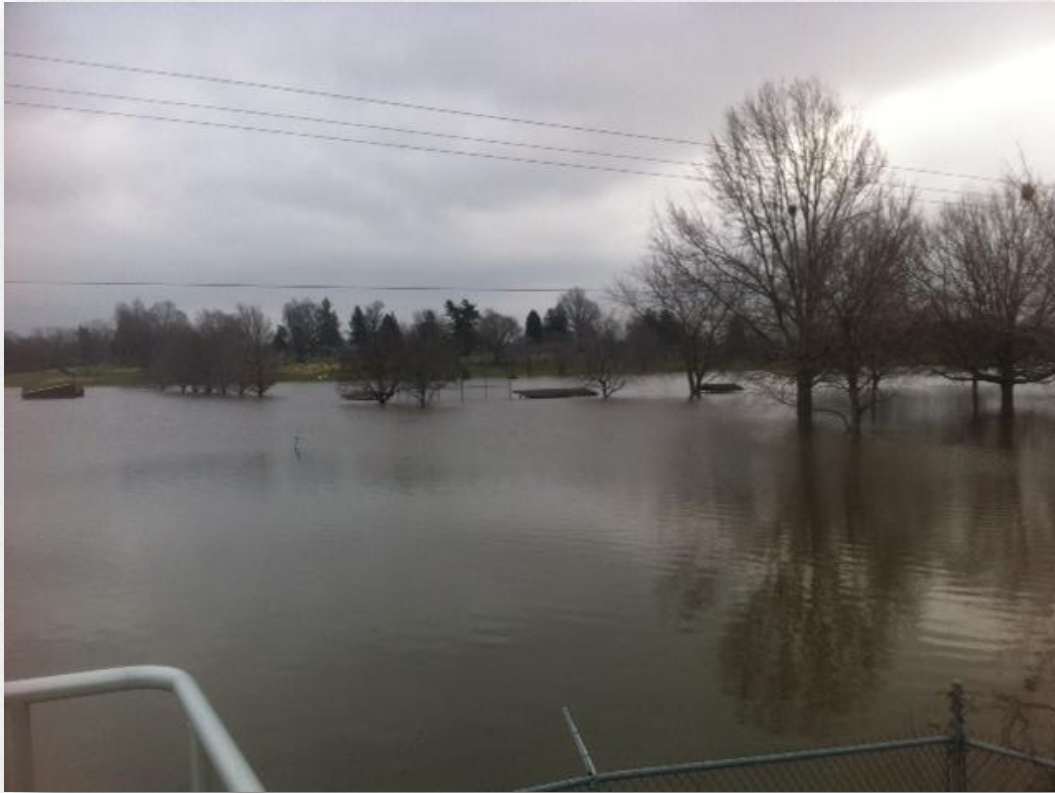
Looking east to park from pump station: WSEL ~546.5
