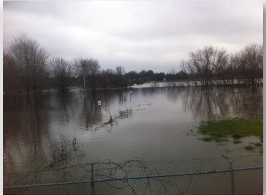
Looking south from pump station
