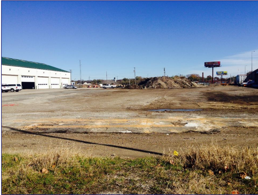
East Site Looking East. Earth Stockpiled in the Background.
