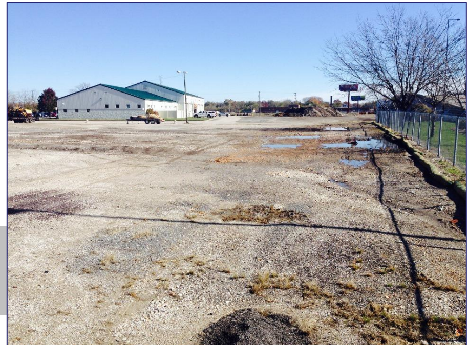
West site looking east prior to construction.
