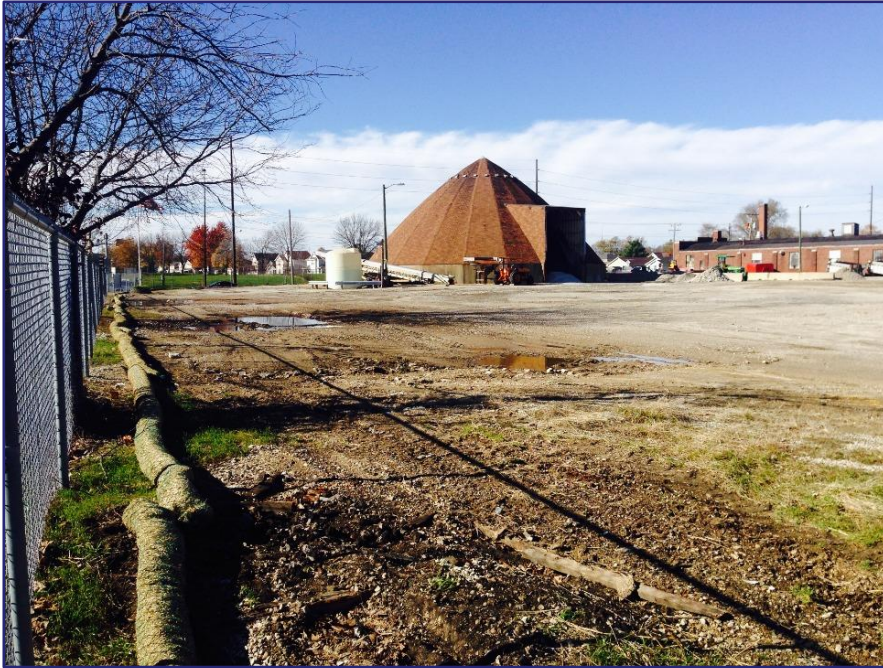
West site looking west prior to construction.
