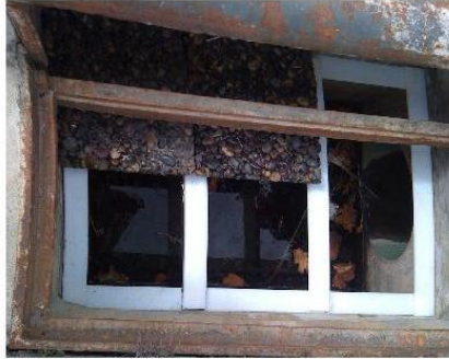
PHOTO OF XERIPAVE TRAY SYSTEM DURING INSTALLATION
