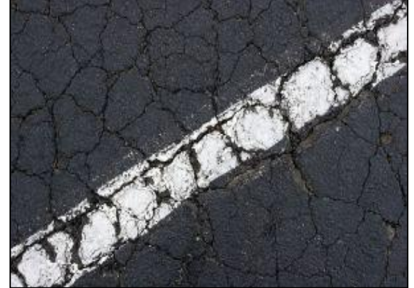
Poor-Mans Permeable Pavement
