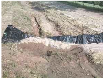
Erosion Control Issues
