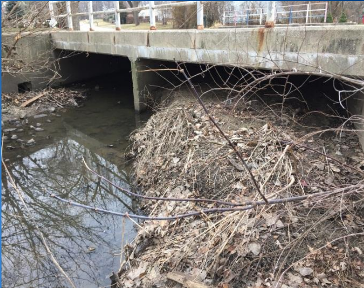
Left: Sediment Build Up at Laporte Ave. Right: Non-Engineered Rip Rap at Laverne Ave.
