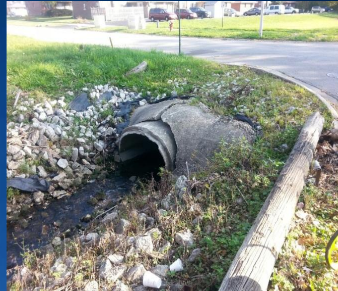
Left: Restrictive 149 th St. Culverts Right: Restrictive Kilpatrick Ave. Culvert at 149 th St.
