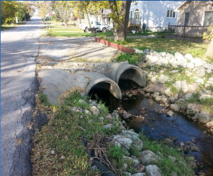
Left: Restrictive 149 th St. Culverts Right: Restrictive Kilpatrick Ave. Culvert at 149 th St.
