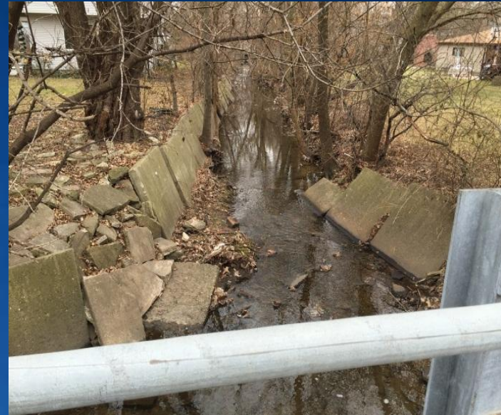
Left: Sediment Build Up at Laporte Ave. Right: Non-Engineered Rip Rap at Laverne Ave.
