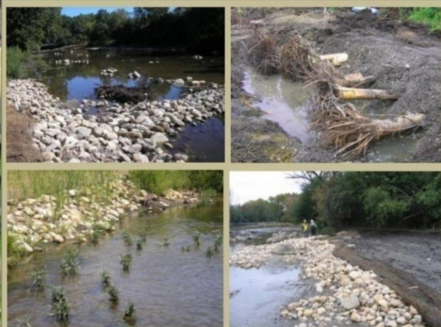
Crenulated bank loading with rock, wood structures and emergent vegetation for improved habitat.
