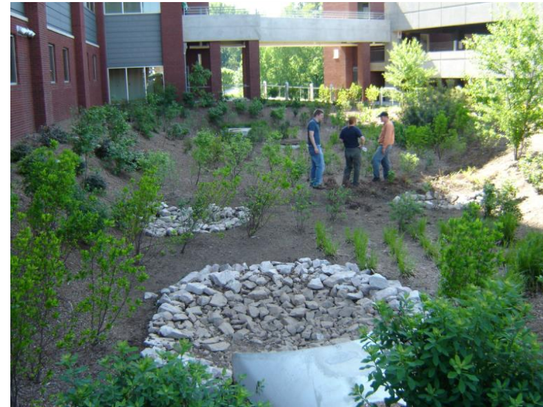
Traditional Bioretention Courtesy: NCDEQ Stormwater BMP Manual
