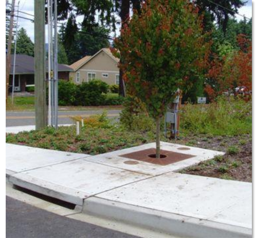
Filterra Offline (with sidewalk inlet flume) Buena Vista - Pierce County, WA
