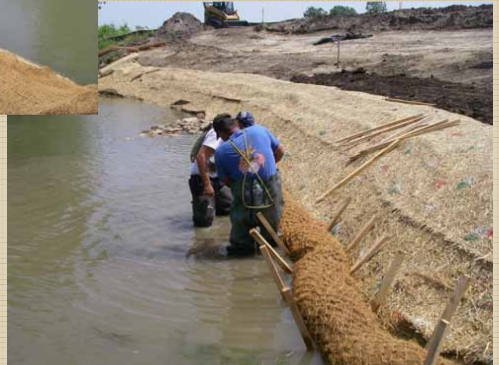
Fiber Roll Installation
