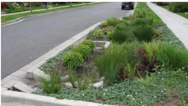
Roadside rain garden/Bumpout
