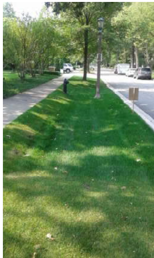
Porous Parkway/ Roadside Swale
