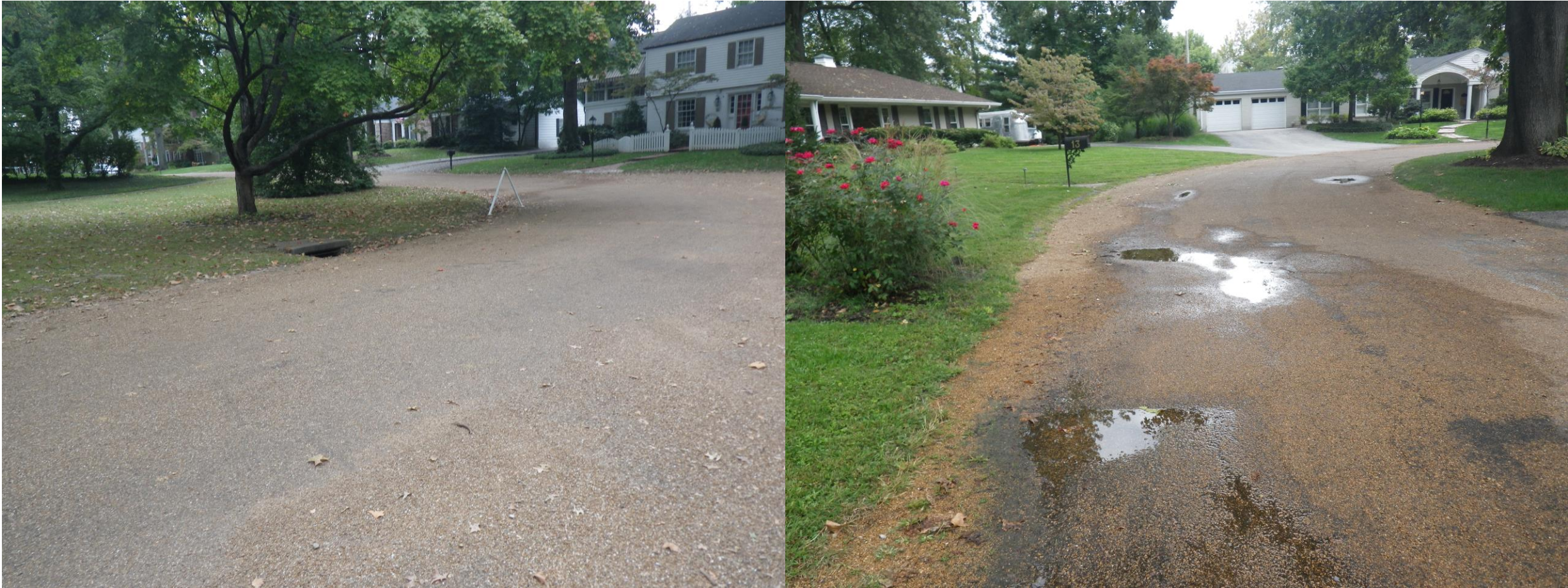
Poor conveyance to inlets
