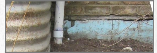
Sill Joint Failure at TF
