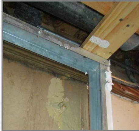
Sill Plate Gap, Fiberglass
