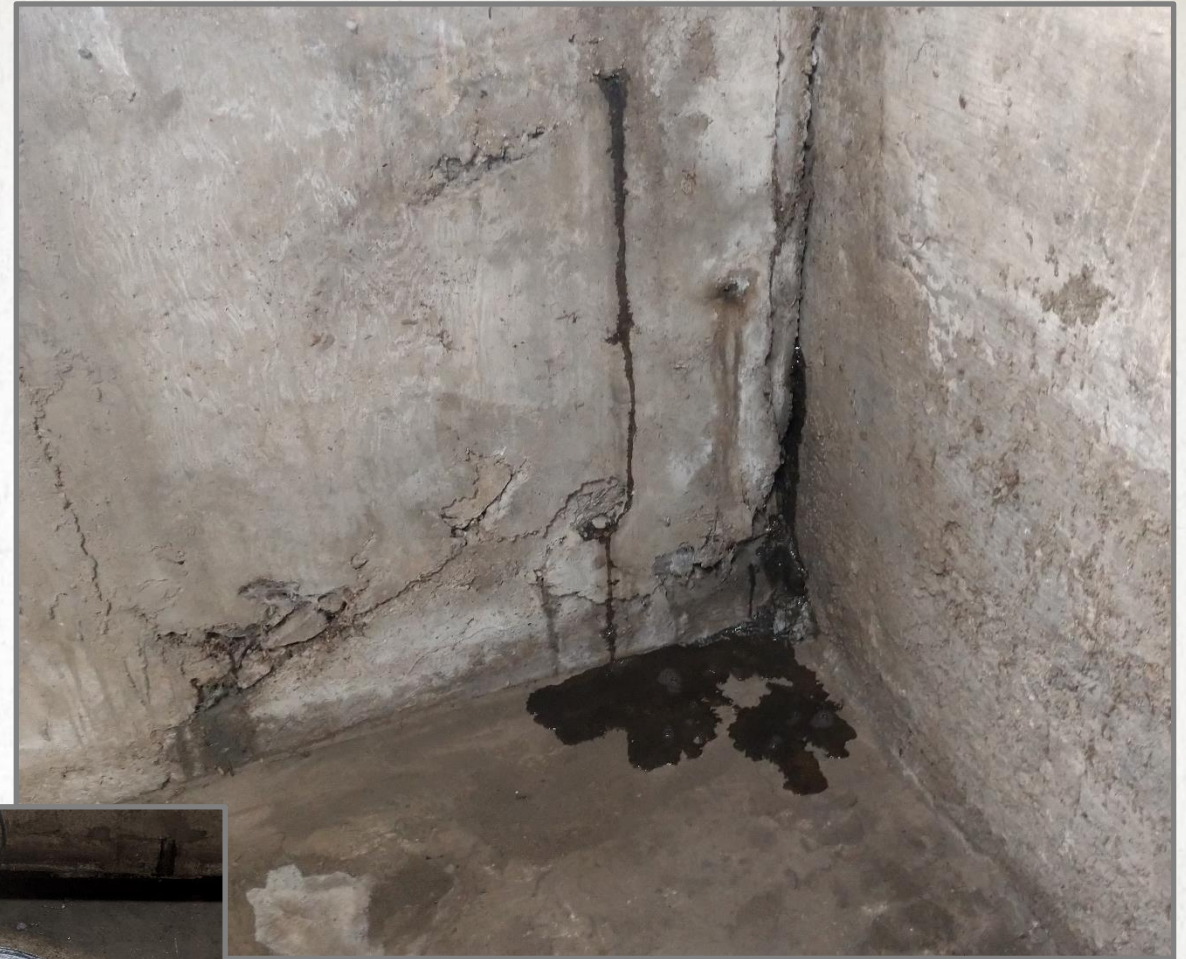
The "Garden Hose" test result – water penetration
