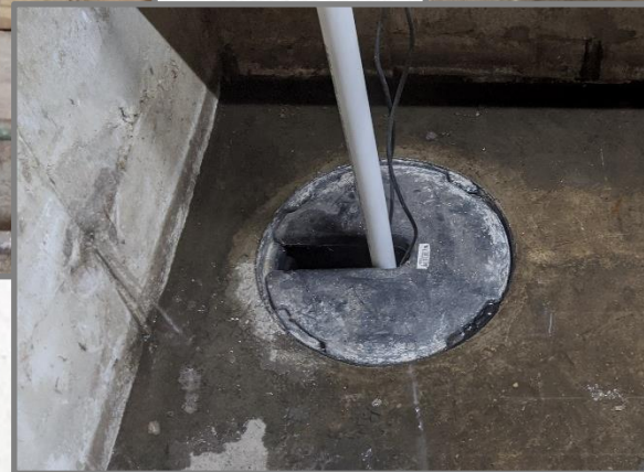
Note storm event water penetration through failed joint or tie
