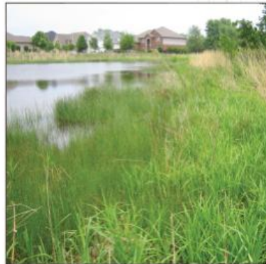
Legend Trail Pond: slope & toe protected with native vegetation
