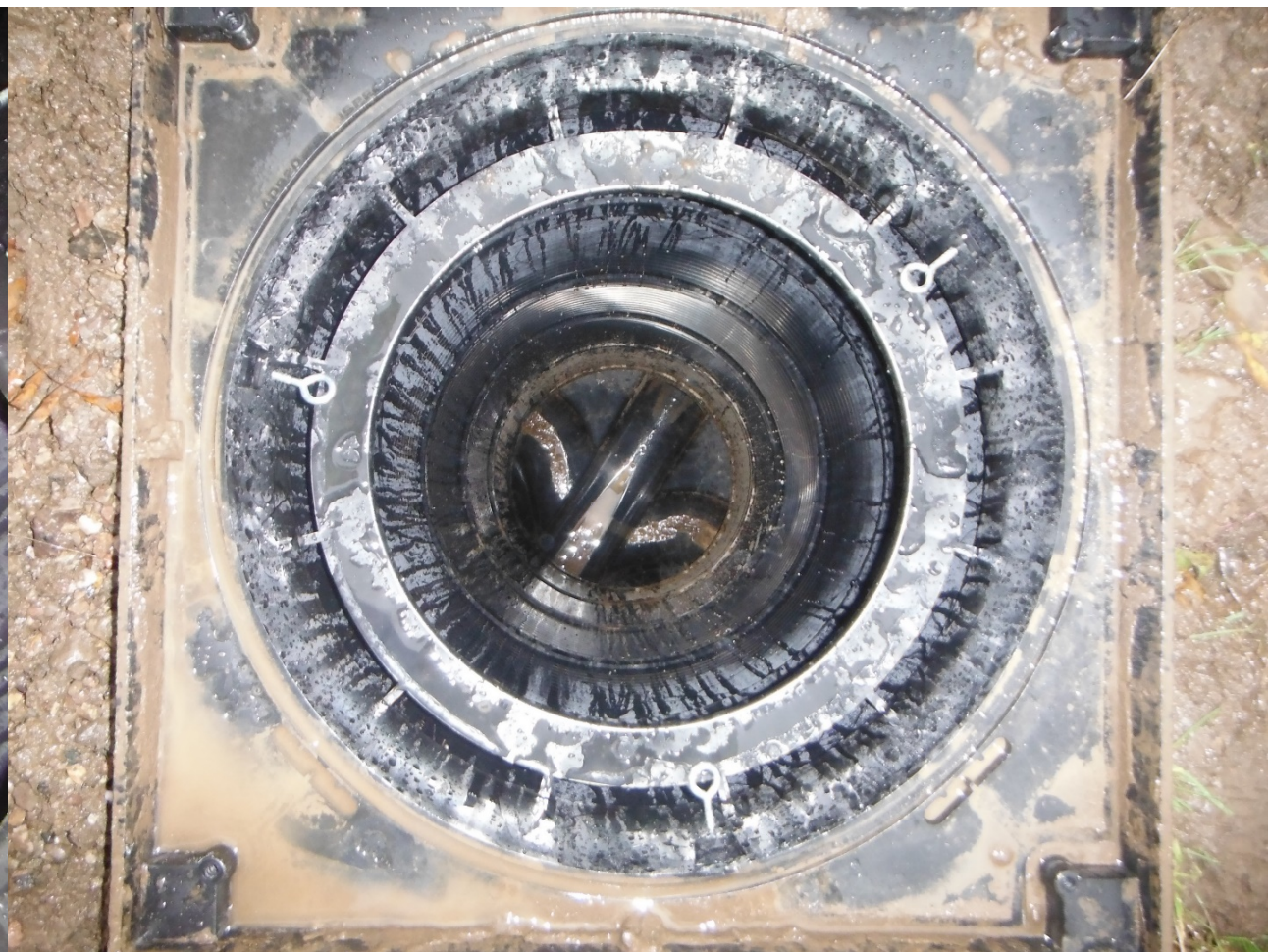
Shows outlet drain - no water flow outwards after 2 hours of rain fall, demonstrating attenuation in action. Some post installation debris visible. This is 80" (2m) down.
