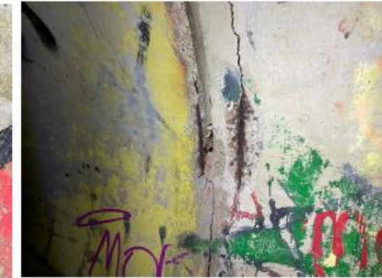
Above: Circumferential cracks at downstream end with exposed rebar.
