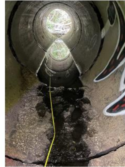
Above: Concrete grout in the invert of the pipe.
