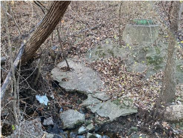
Upstream End: Deterioration of grouted channel & slope above culvert inlets. Overgrowth and debris.
