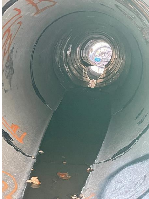
Culvert pipes are settling at both ends
