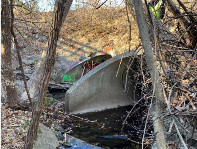
Upstream End: Deterioration of grouted channel & slope above culvert inlets. Overgrowth and debris.
