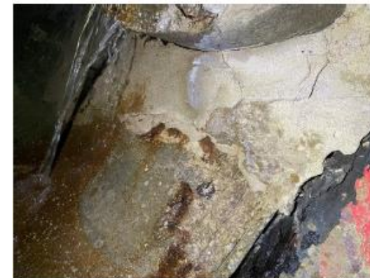
Above: Pipe wall condition below 36 inch RCP penetration.
