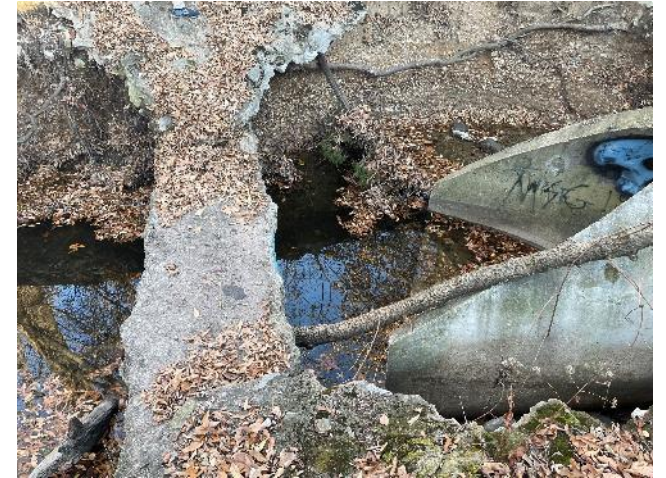
Downstream End: Channel Incising, bank scour, exposed sanitary sewer, & flared end settling/disconnected
