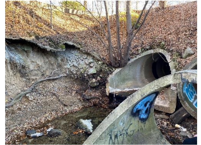
Downstream End: Channel Incising, bank scour, exposed sanitary sewer, & flared end settling/disconnected
