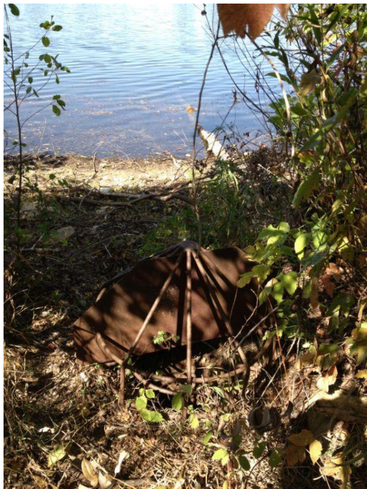
Corroded Drop Inlet CMP
