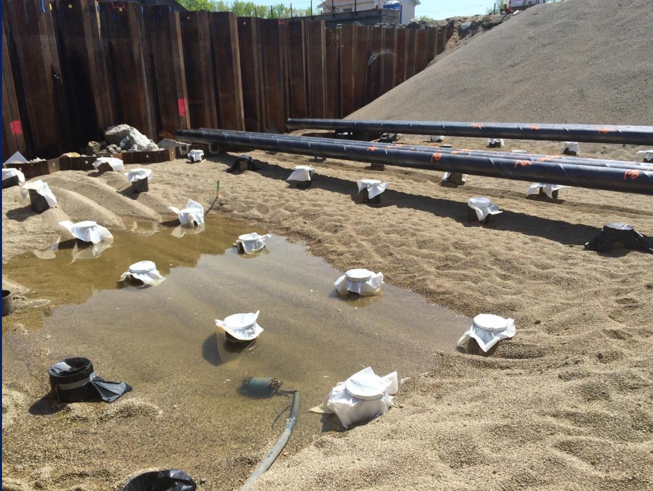
■ Gate Phase 1 Metal Shell Piles
