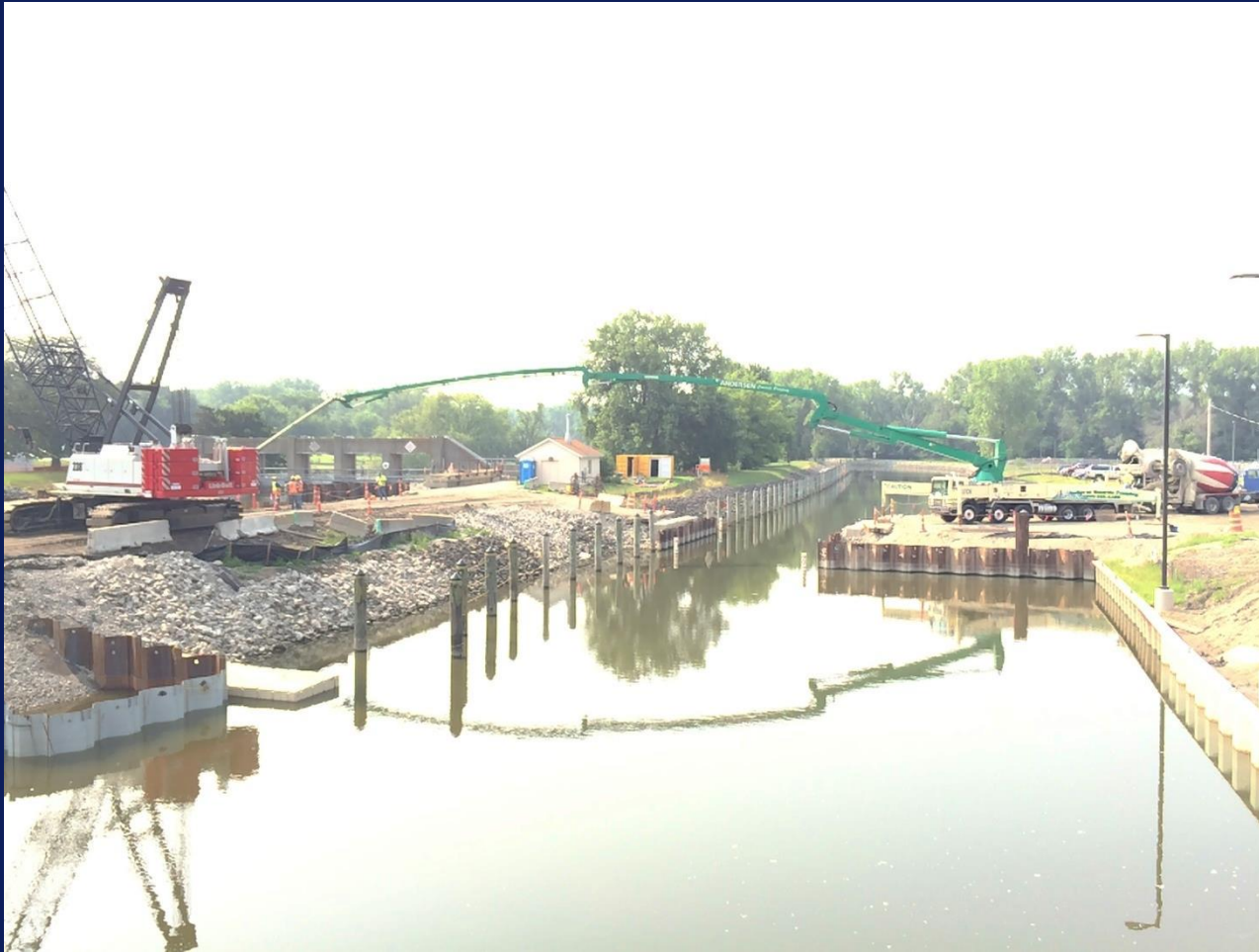
■ Phase 1 Base Slab Concrete Placement
