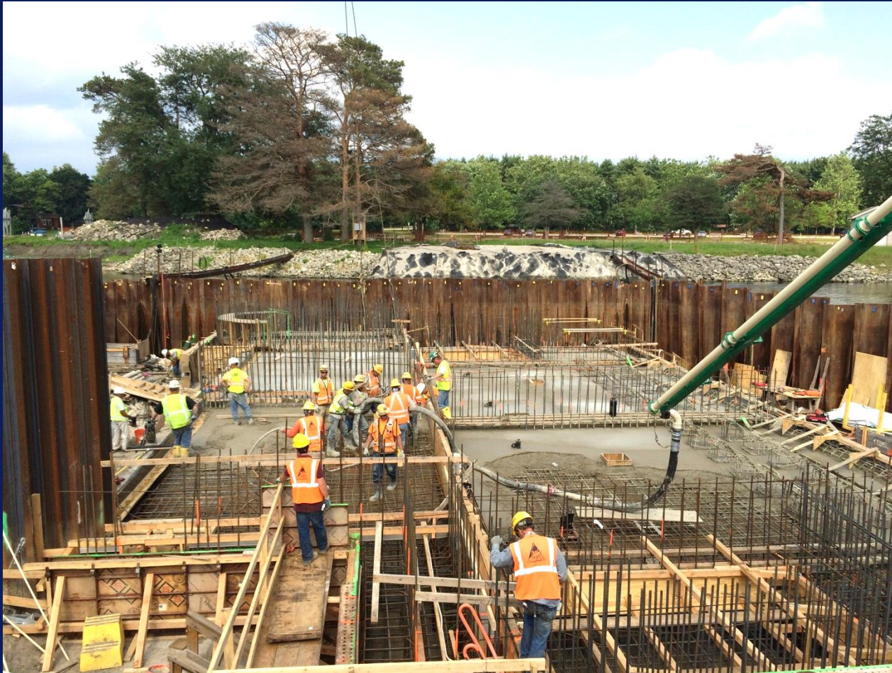
■ Phase 1 Base Slab Concrete Placement
