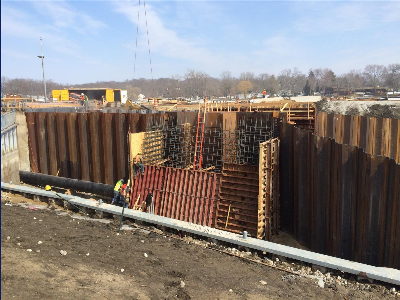
■ Monolith Formwork being assembled
