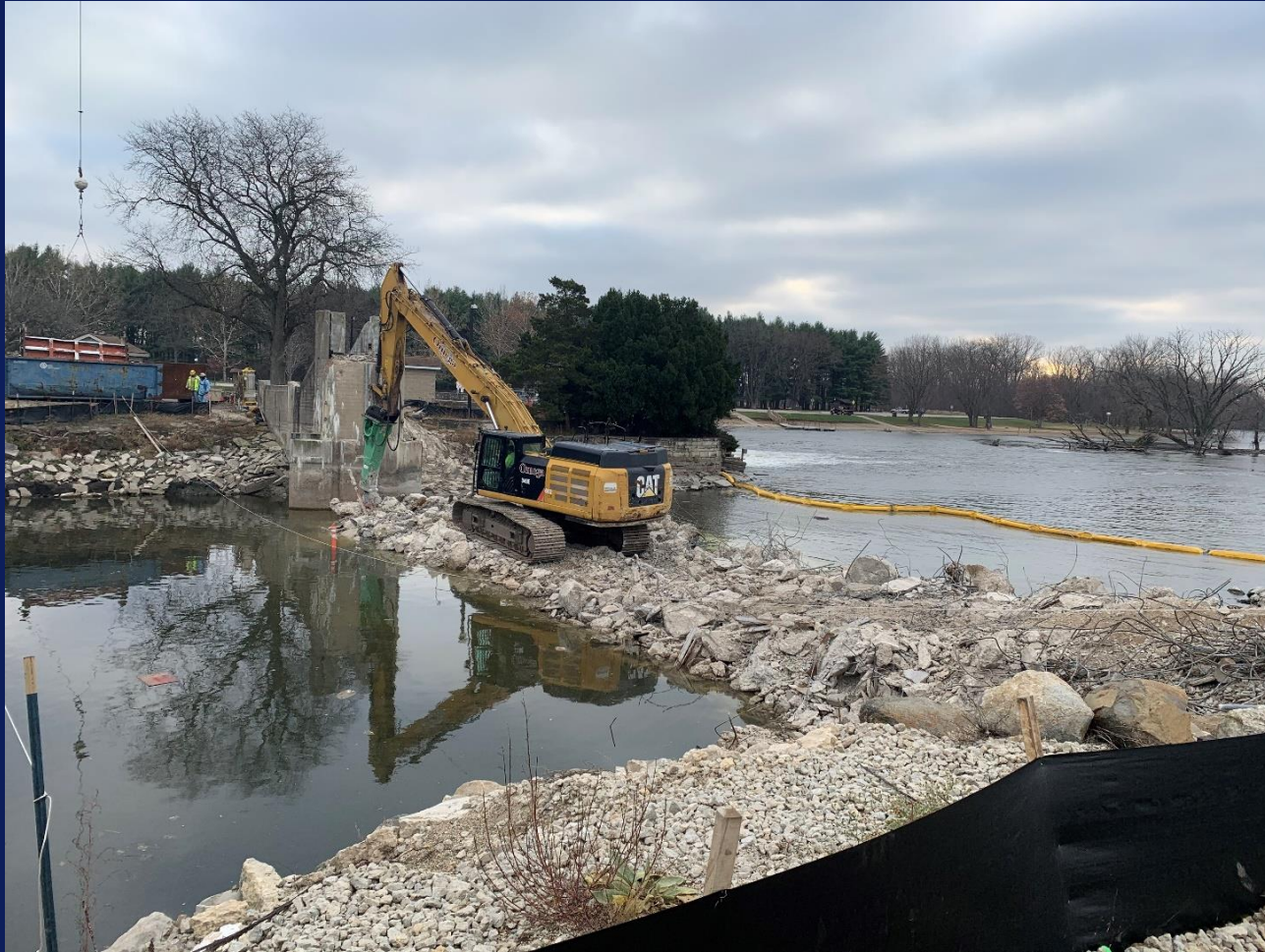
Demolition of Existing Dam Structure
