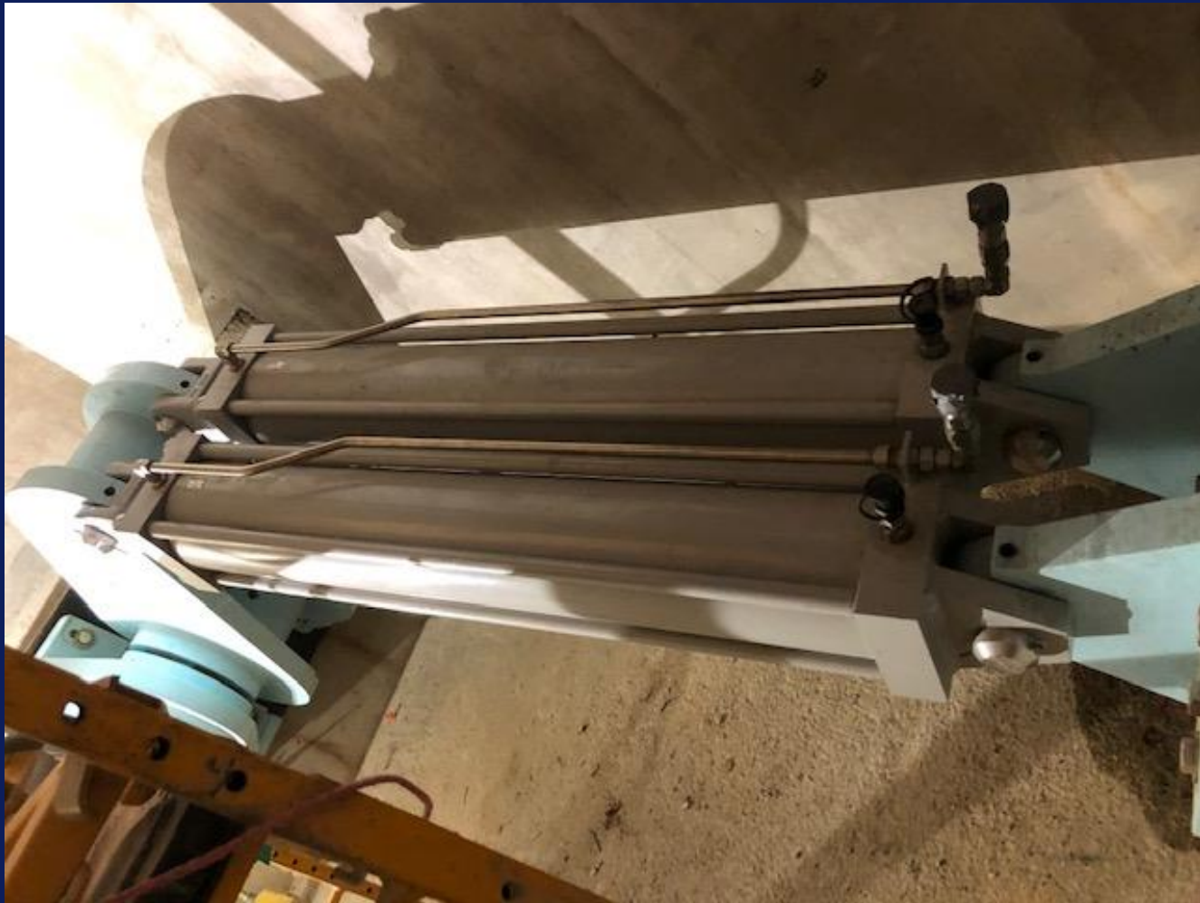
Hydraulic cylinders in place in vaults 1 & 2
