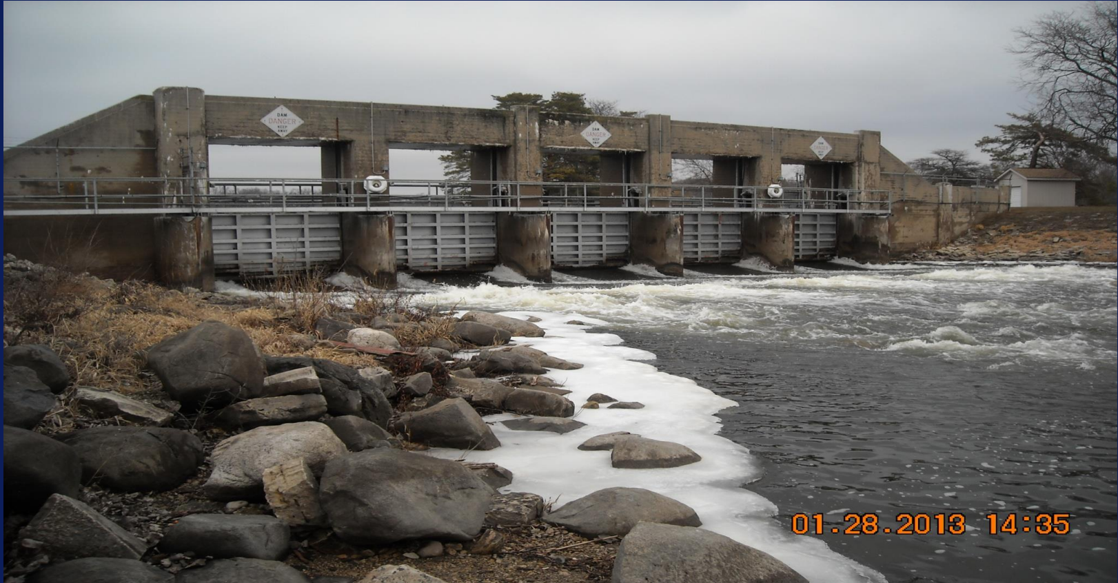
Existing Structure with 5 Vertical Roller Gates
