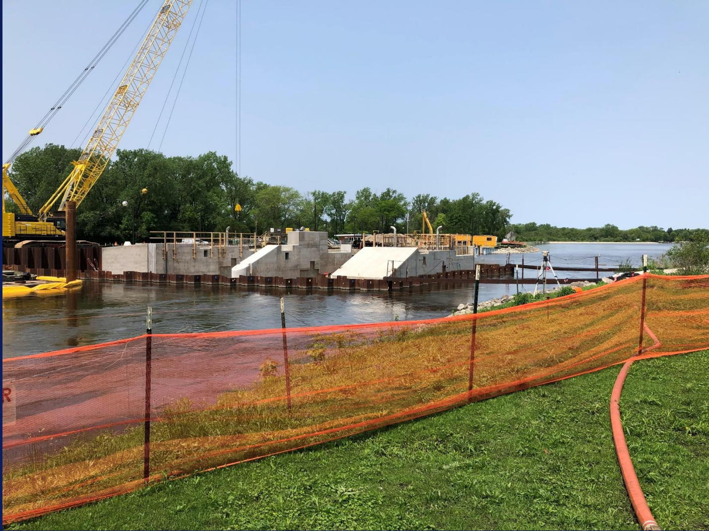
Concrete forms stripped from vaults
