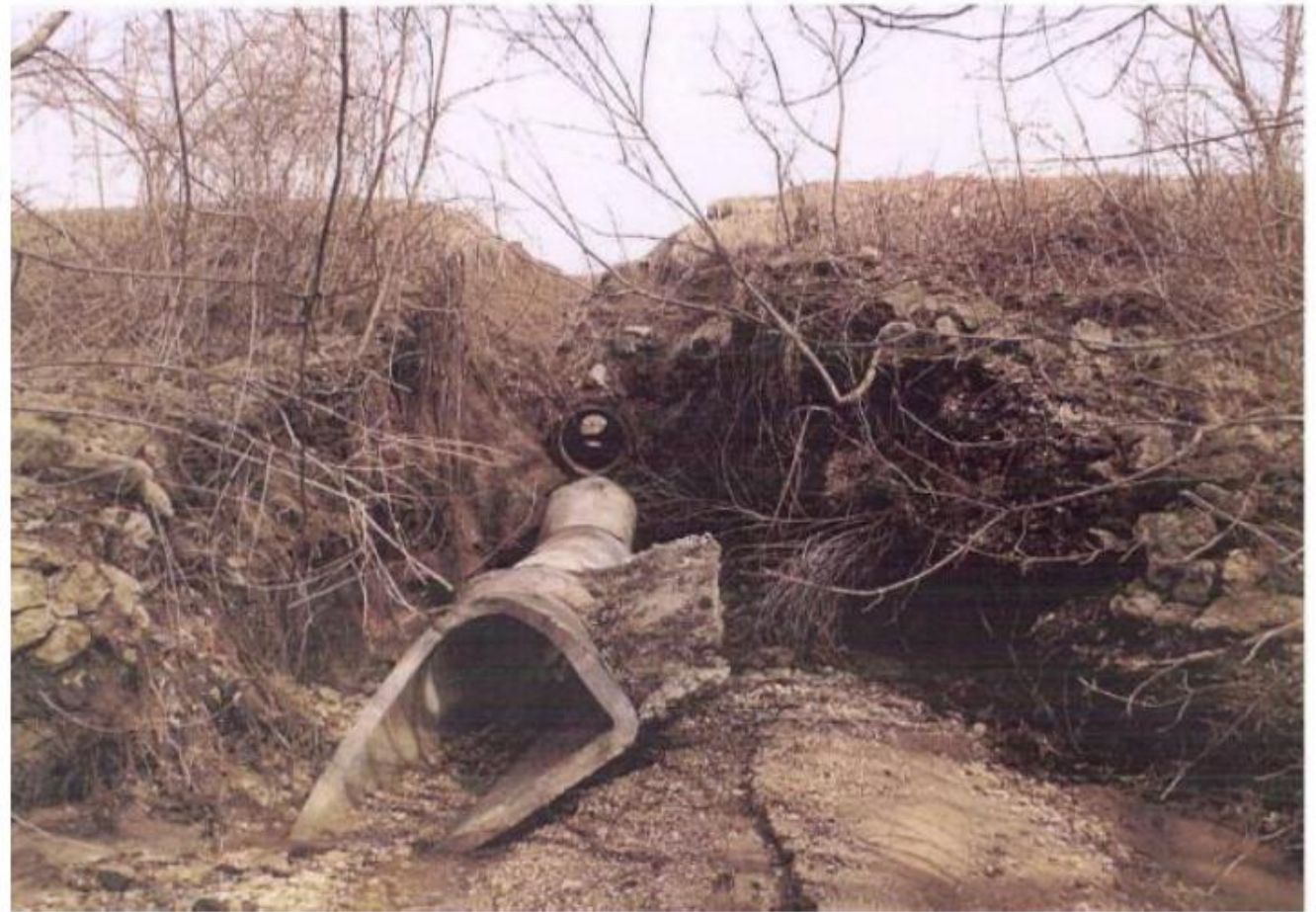
Figure 17. View looking north from downstream end of outlet area of SWM detention pond 1 showing erosion over top of outlet culvert and erosion below outlet. (Photo taken in April 2008.)
