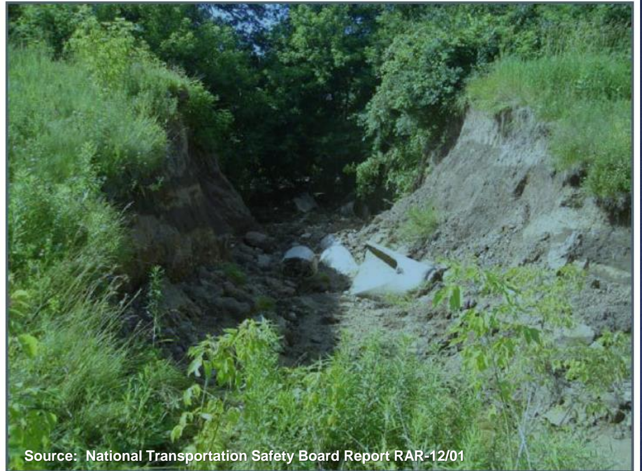
Figure 16. Postaccident photograph showing breach in SWM pond 1 as viewed from inside pond looking south.
