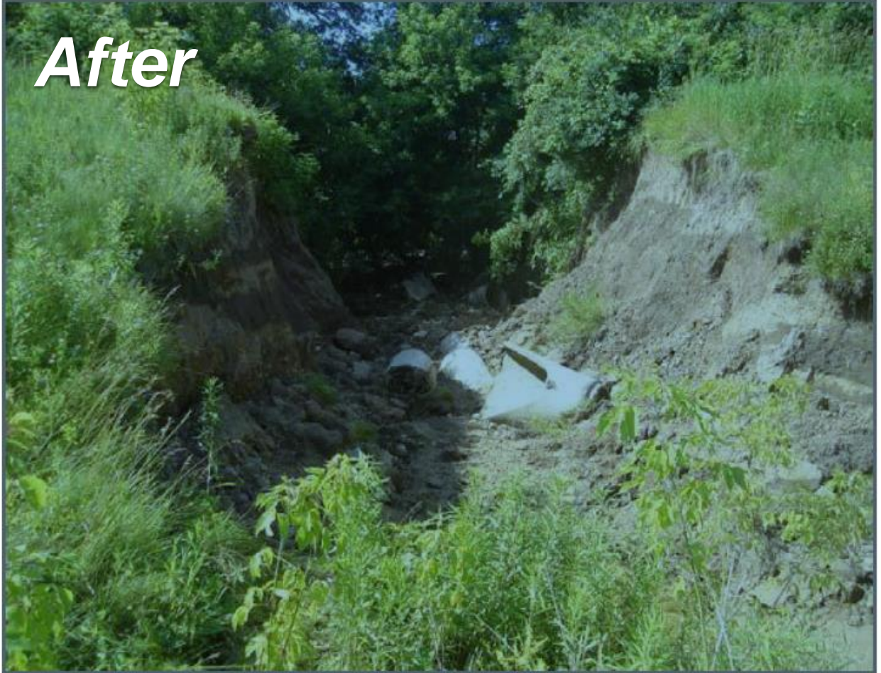
Figure 16. Postaccident photograph showing breach in SWM pond 1 as viewed from inside pond looking south.
