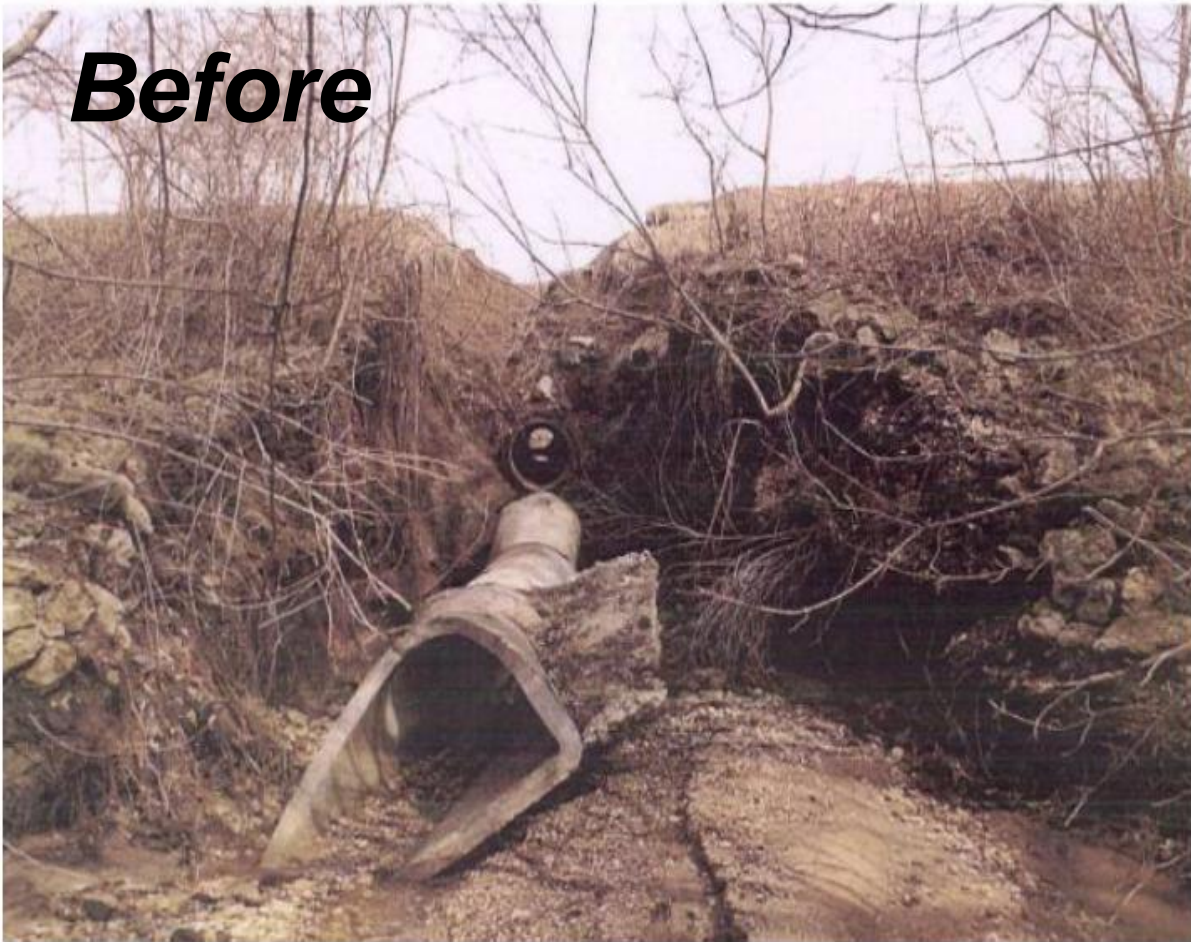
Figure 17. View looking north from downstream end of outlet area of SWM detention pond 1 showing erosion over top of outlet culvert and erosion below outlet. (Photo taken in April 2008.)
