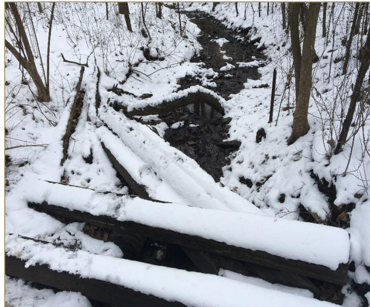
Blocked Channel & Failing Bridge
