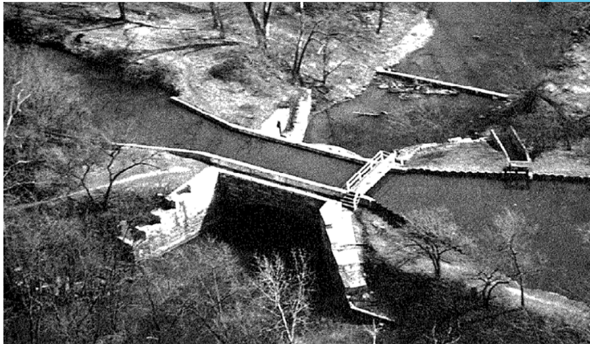
Photograph of the Nettle Creek Aqueduct, taken circa 1974.
