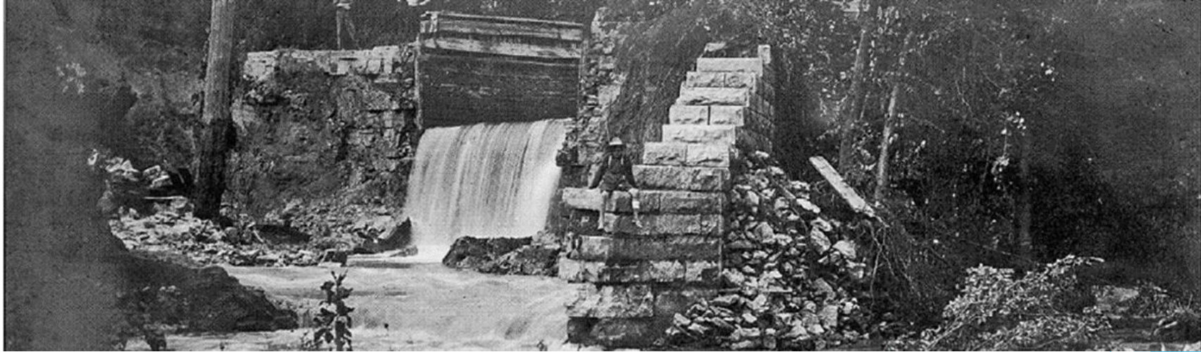
Nettle Creek Aqueduct after a break in the canal in the spring of 1910.
