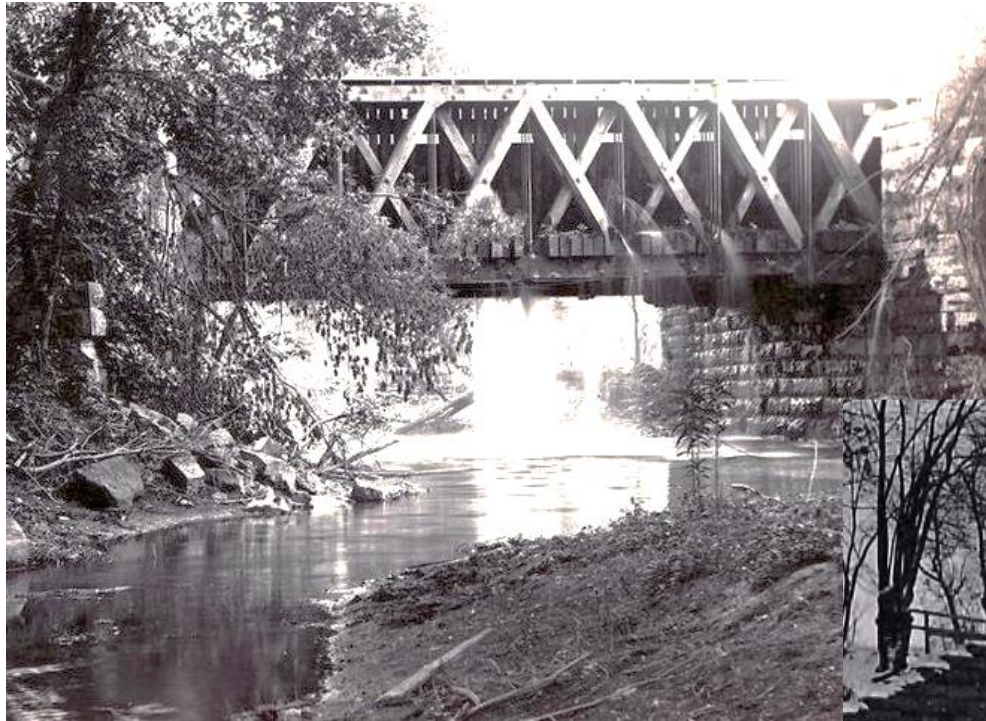
Photograph of the Nettle Creek Aqueduct, likely dating from the late nineteenth century.
