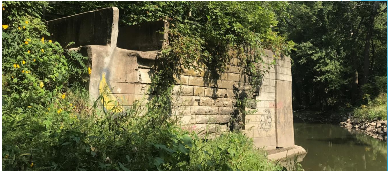
2020 condition of Nettle Creek Aqueduct (Wing-wall) .
