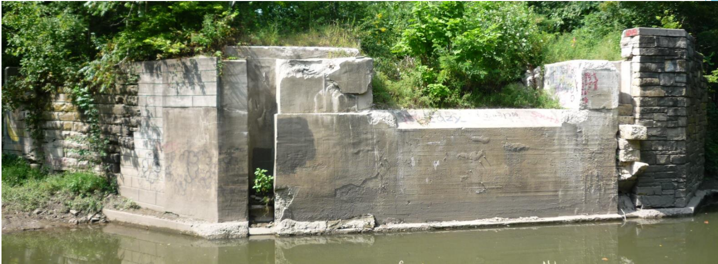
2020 condition of Nettle Creek Aqueduct.
