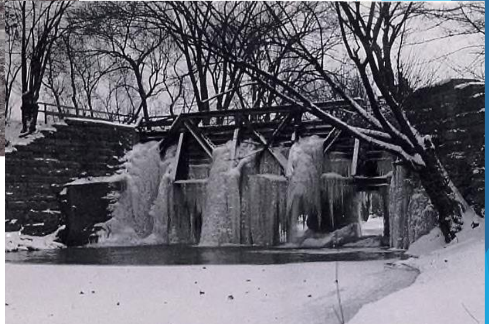
Nettle Creek Aqueduct showing the steel-frame structure that was installed in 1910.
