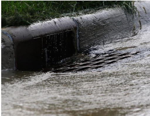
Storm Sewers, Inlets, & Swales 10-year capacity (min.)
