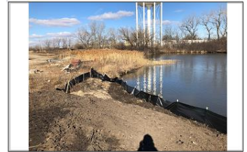
Silt fence is in good condition
