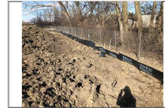
Silt fence is in good condition
