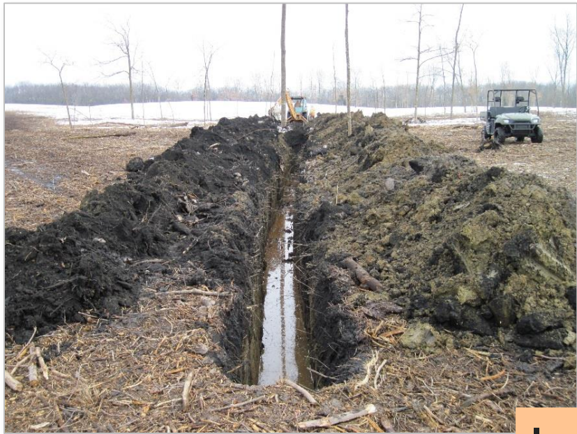
Drain tile removal
