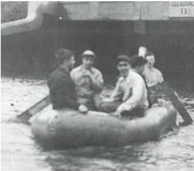
Flossmoor Rd. Viaduct - 1951
