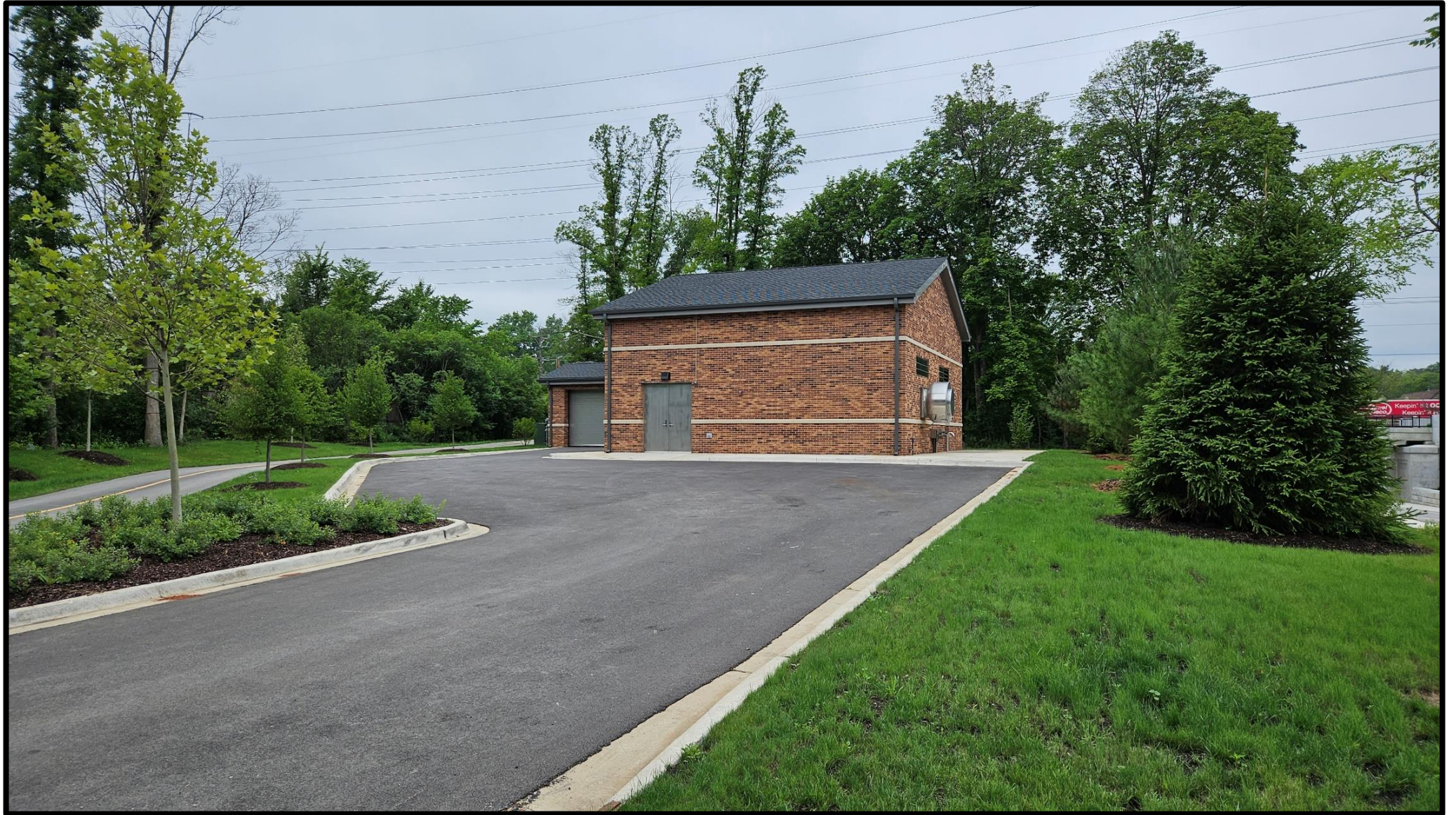
Pump Station 38 Site and Front of Building Exterior
