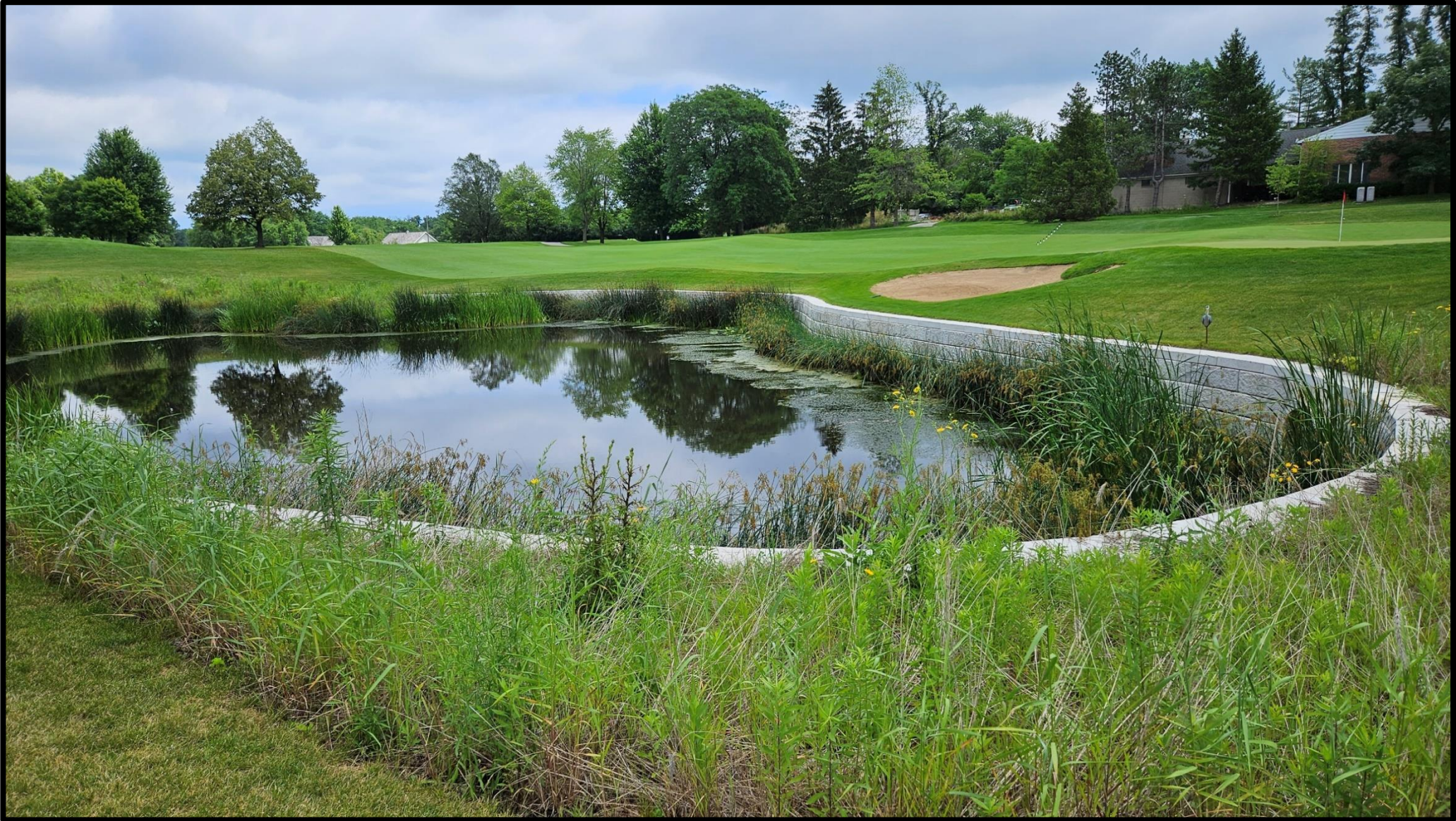
Deerpath Golf Course West Detention Pond with “Serpentine” Retaining Wall
