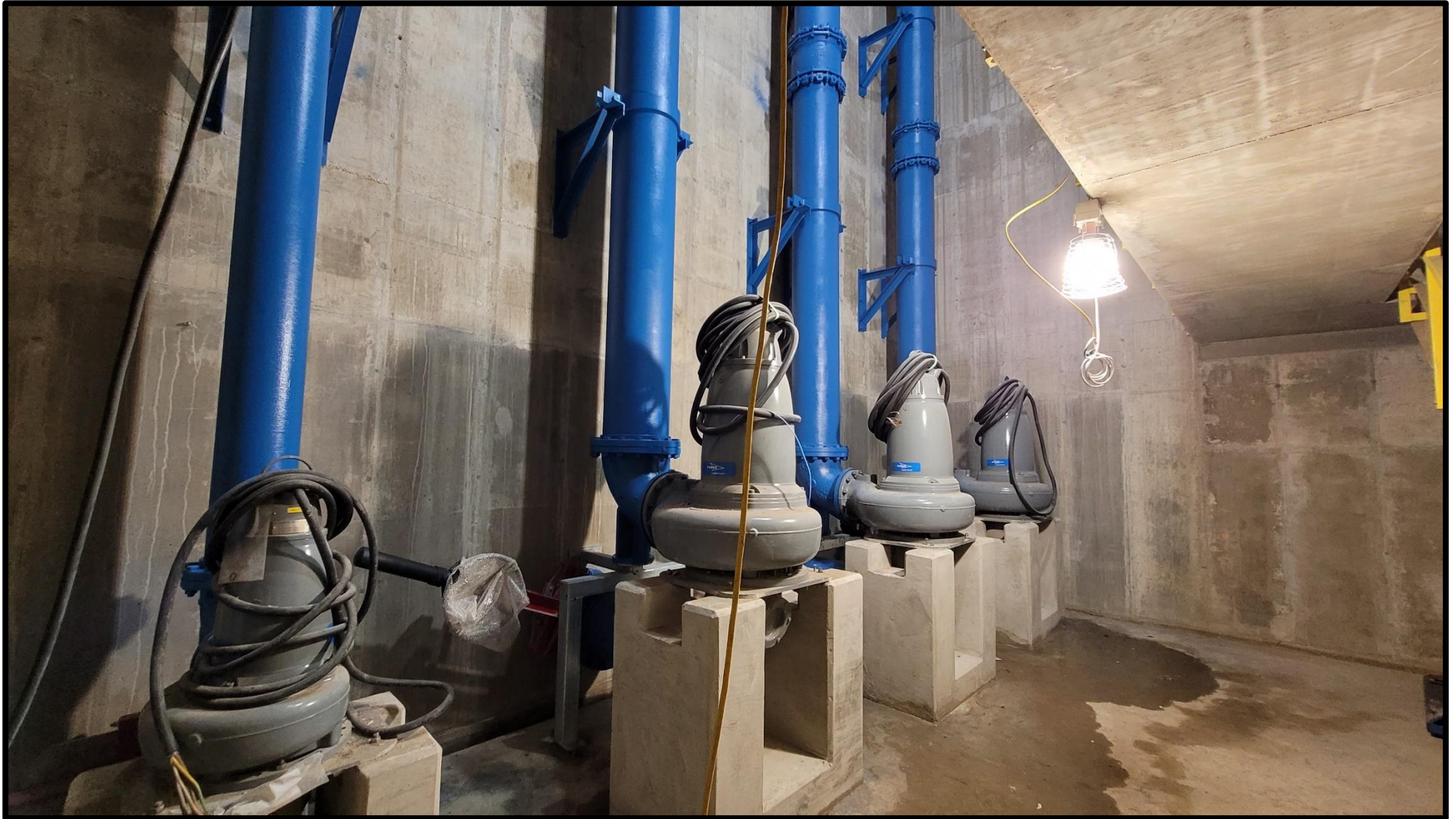
Dry Well with Pumps Partially Installed 3 – 5,700 gpm and 1 – 1,900 gpm
