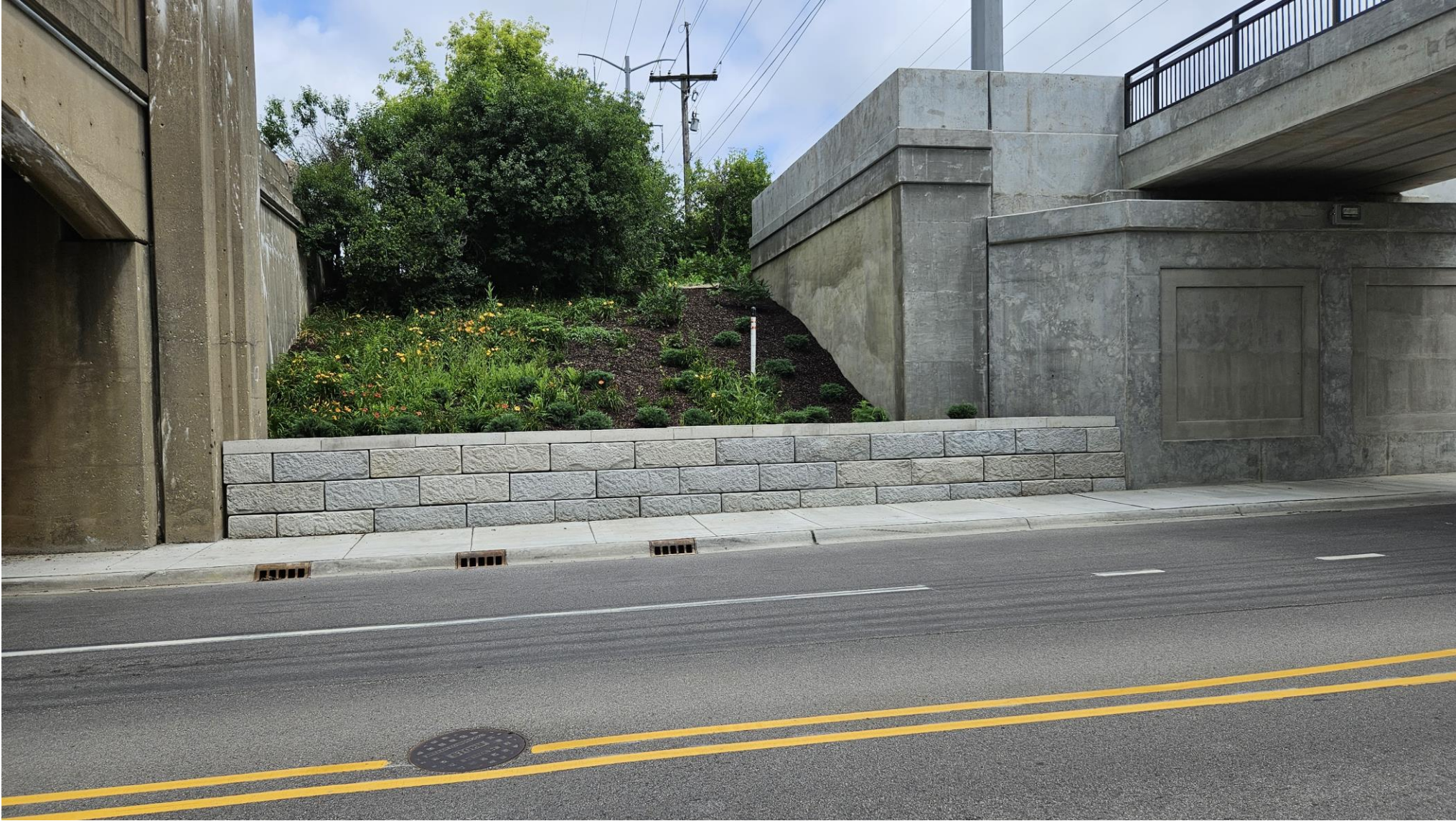
New Retaining Wall built taller to ease slope
