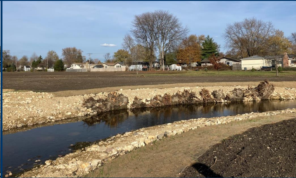
Carol Stream Project Streambank Stabilization
